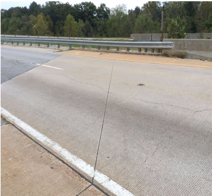
PHOTO 1 Description Sealable cracking at both slabs.
