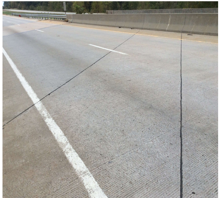
PHOTO 2 Description Deck has sealable cracking in all spans.
