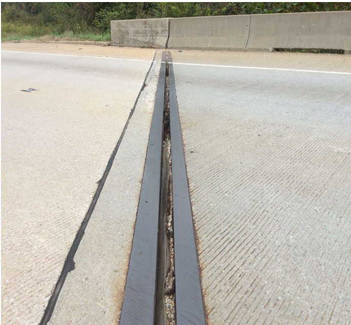
PHOTO 1 Description Compression joint seals at the abutments and the poured joint material at the intermediate expansion joints have deteriorated and are failing.
