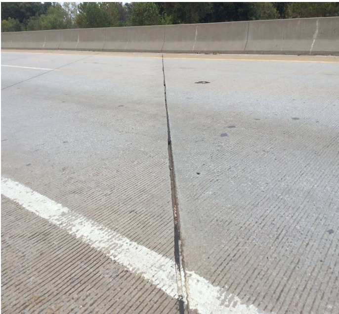
PHOTO 1 Description The poured saw joint seals are deteriorated and missing in locations.
